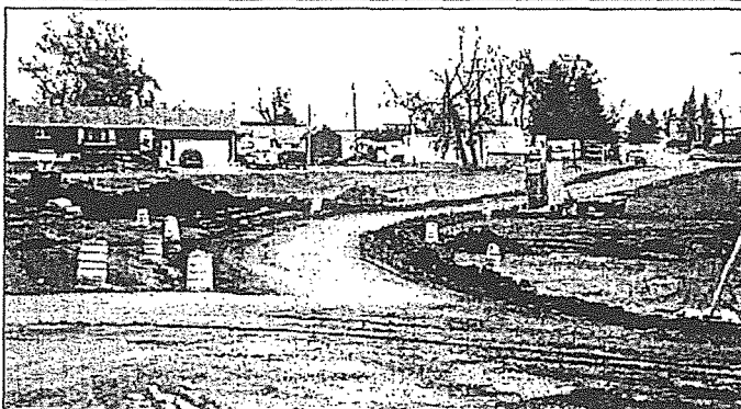
A temporary road from Borchardt Ave. to Stewart Ave, was built as a detour for folks travelling south of Underwood's Borchardt Ave. Photo by Suzanne Werre
