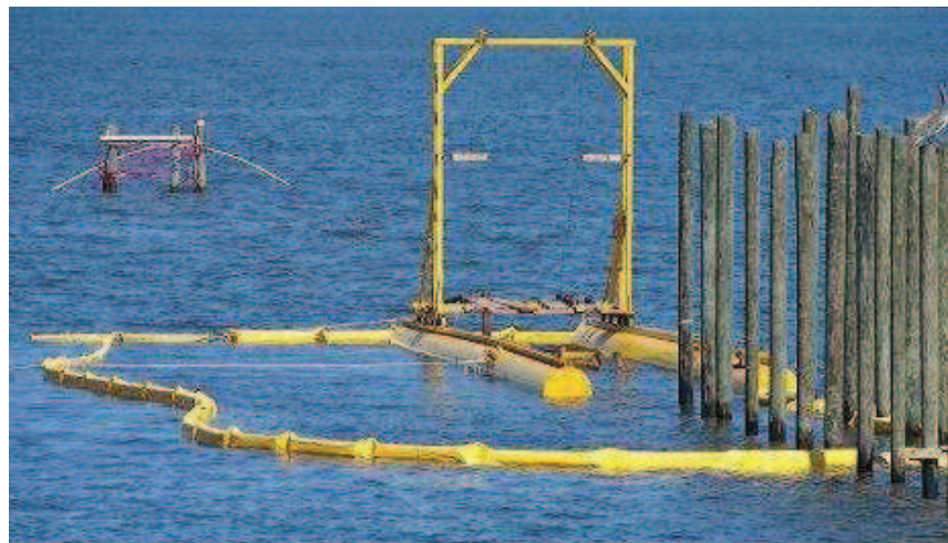
Type 1 Silt Barrier used on a pile driving on Intercoastal - Florida USA
