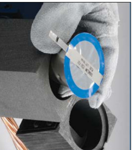
Figure 5. Installation of CadWeld Plus charge
