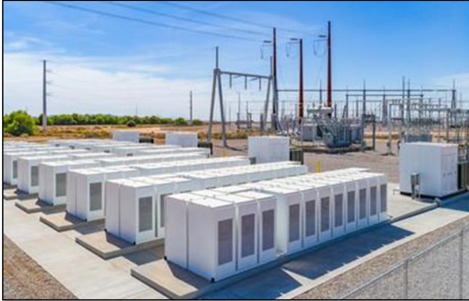
Image 7-2. Example of a self-contained energy storage system cabinet.
