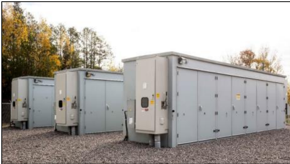
Image 7-1. Example of a self-contained energy storage system cabinet.
