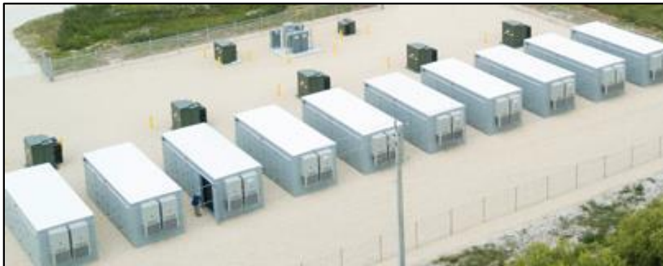
Image 7-3. Example of a self-contained energy storage system cabinet.
