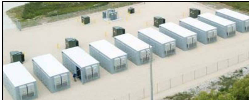
Figure 2c. Example self-contained energy storage system cabinet.
