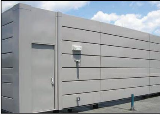
Figure 3b. Example of sound barrier (IAC Acoustics 2023).
