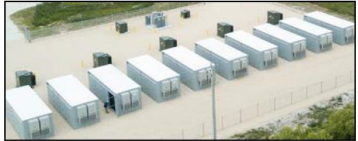
Figure 2c. Example self-contained energy storage system cabinet.
