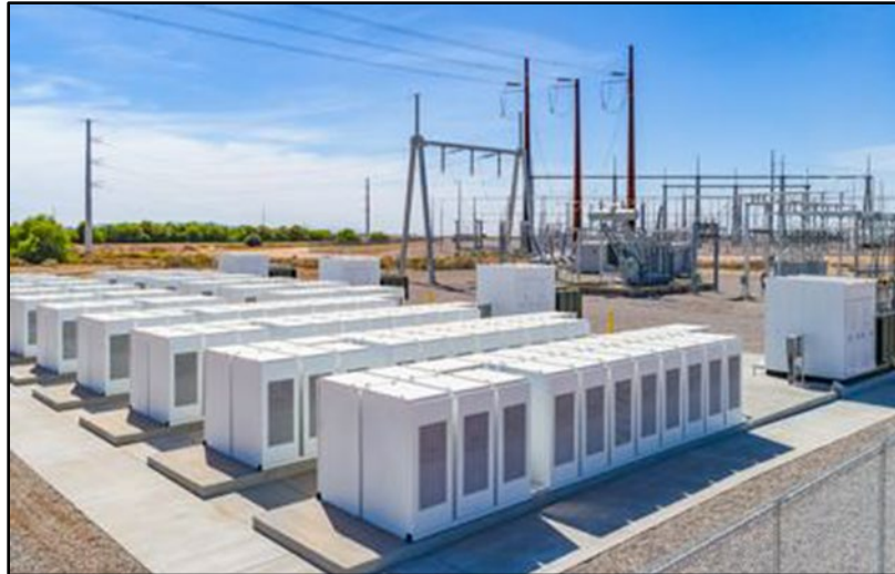
Figure 2b. Example self-contained energy storage system cabinet.
