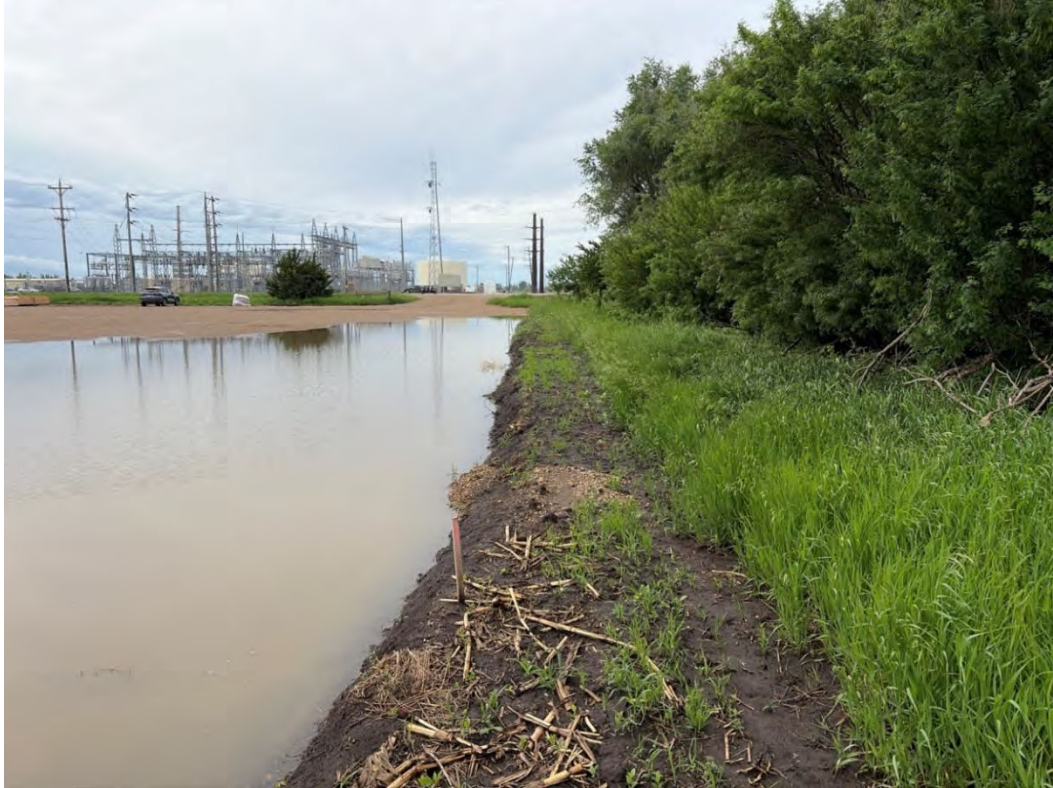
Photograph 3. Overview of Project APE, facing south. NorthWestern equipment laydown area in foreground and substation in background.
