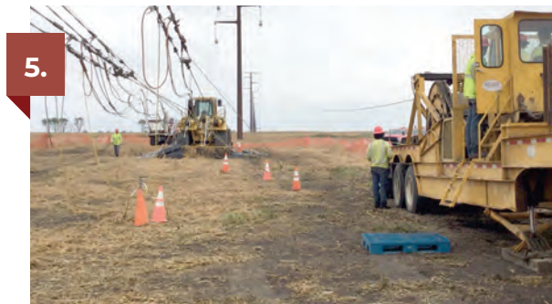
Conductor stringing
