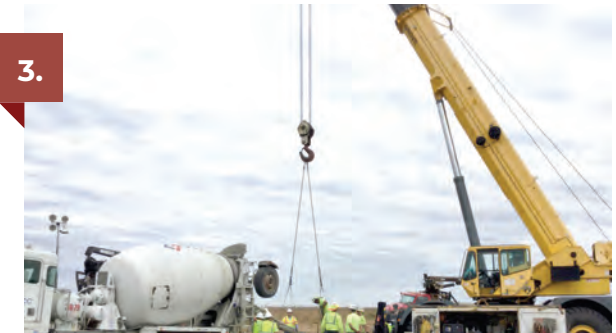
Foundation drilling and pouring
