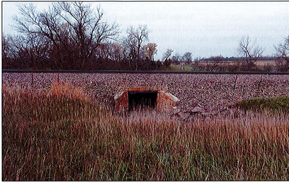
Figure 14. View of MH00002387 facing west. J. Larson 10/27/2016.
