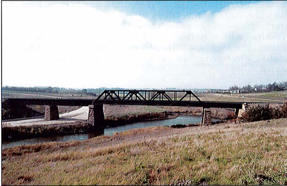
Figure 7. View of MH00000902 facing west-southwest. J. Larson 10/27/2016.
