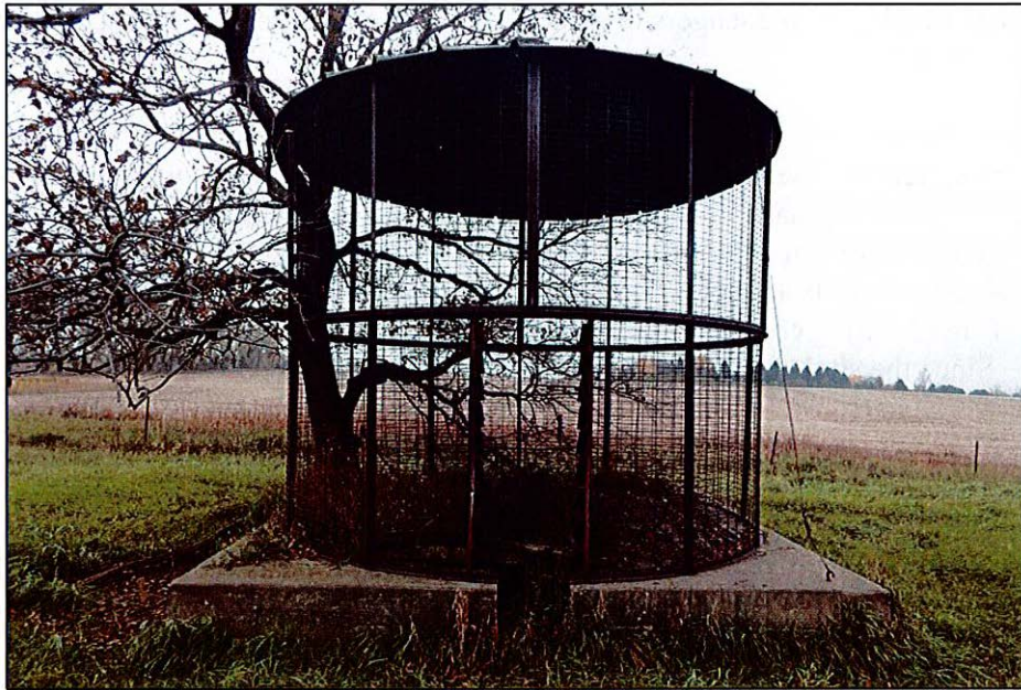
Figure 13. View of MH00002386 facing south. J. Larson 10/27/2016.
