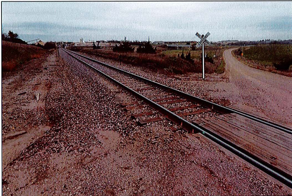
Figure 12. View of 39MH2013 where it crosses 259th Street, facing southwest. Note wood slats used for railroad crossing. Photograph taken at south end of site. J. Larson 10/25/2016.
