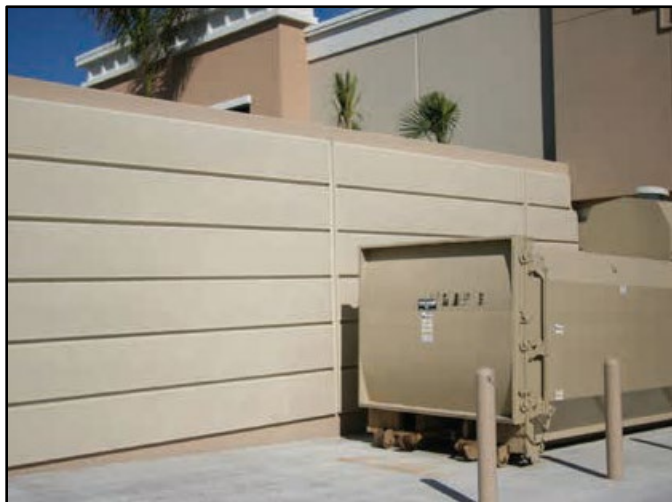
Figure 3a. Example of sound barrier (IAC Acoustics 2023).
