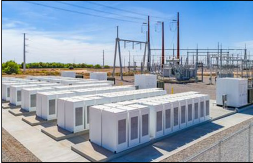
Figure 2b. Example self-contained energy storage system cabinet.
