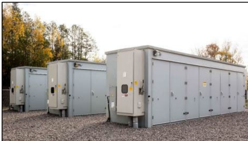
Figure 2a. Example self-contained energy storage system cabinet.
