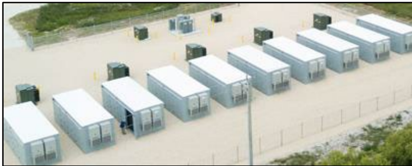
Figure 2c. Example self-contained energy storage system cabinet.
