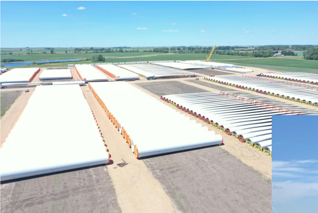
Construction laydown yard
