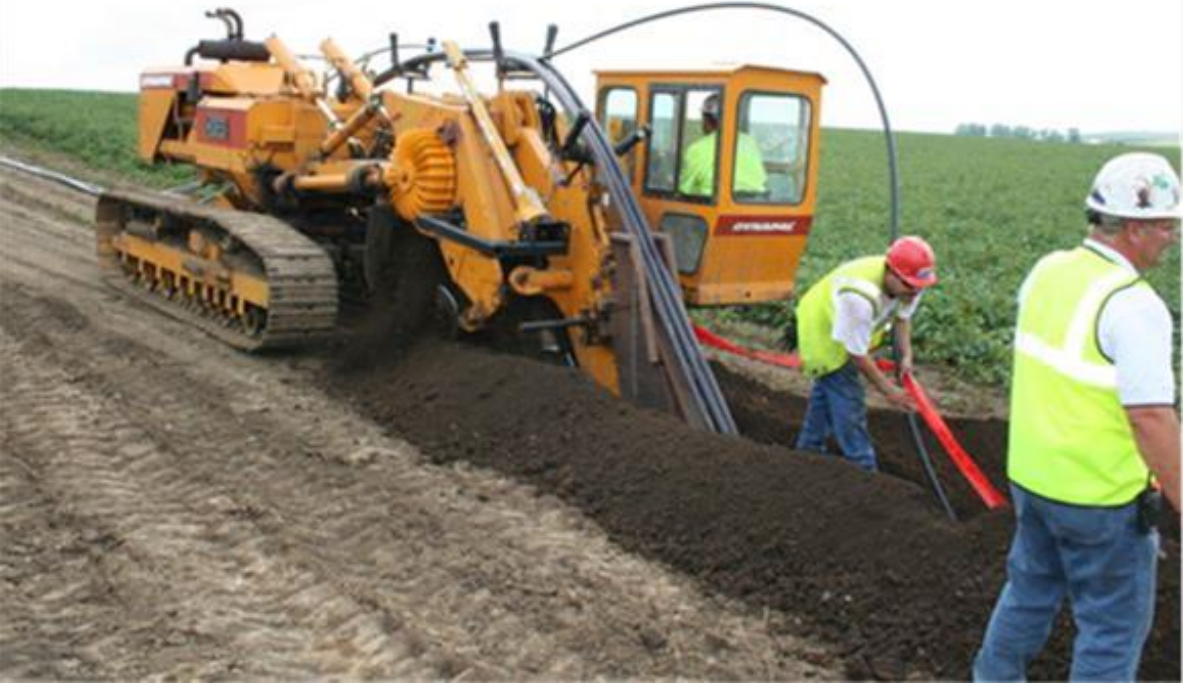
Underground collector circuit and fiber optic cable installation.
