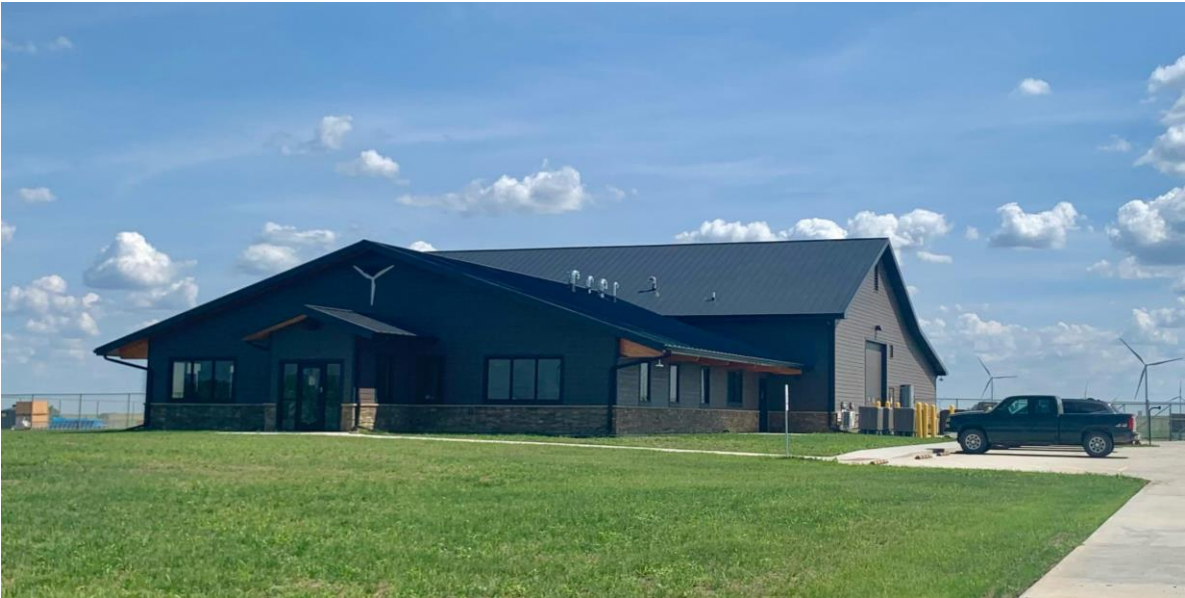
Operations & Maintenance Building (North Deuel Wind Farm).
