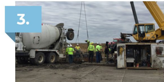
Foundation Drilling & Pouring
