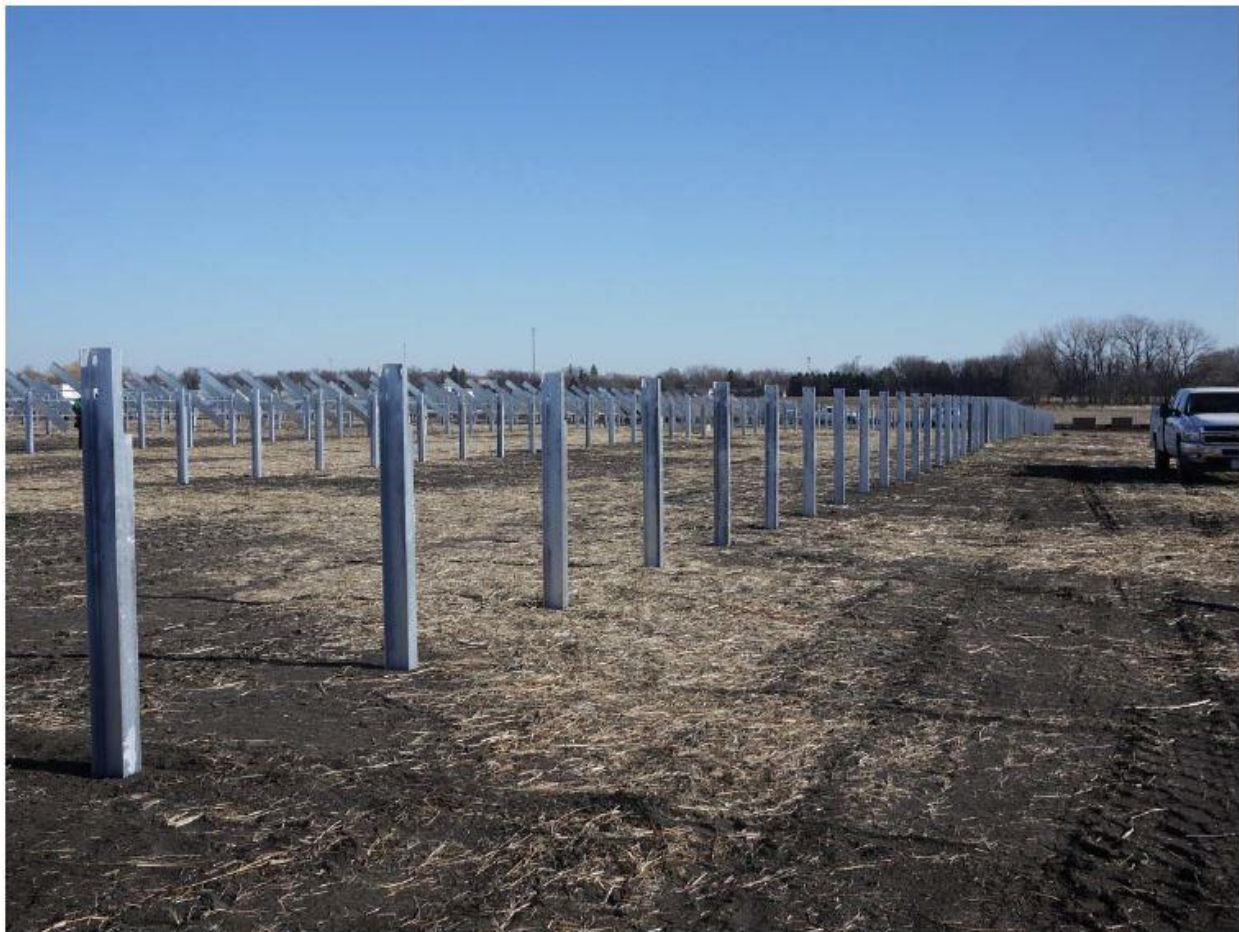
Image 3 Standard Steel Pier Foundations
