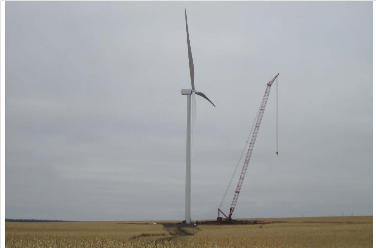
Photo: Wind tower construction west of Waverly
