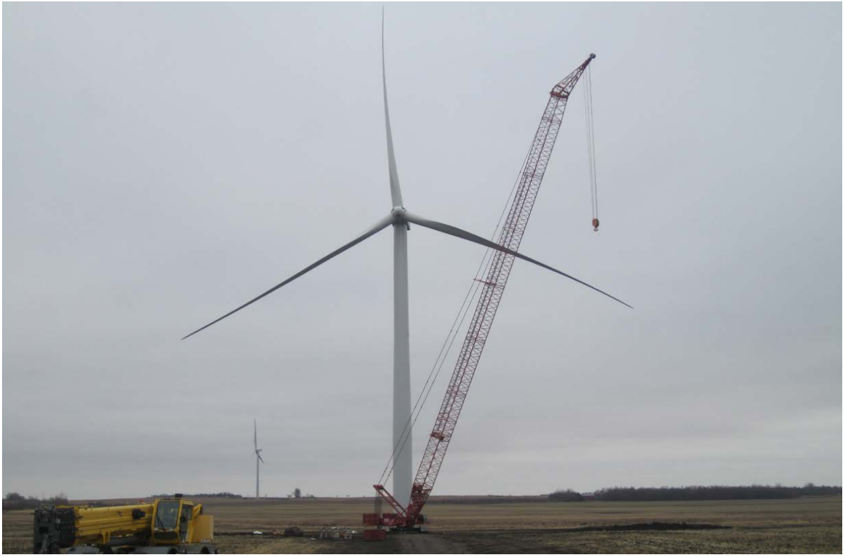
Photo: Wind tower construction west of Waverly.
