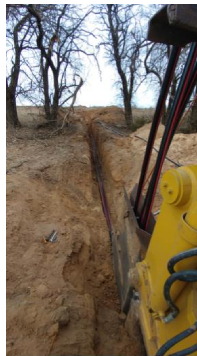
34.5- kV underground trench, approximately 42" deep. Slide 21
