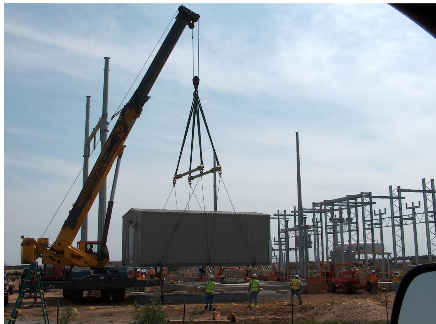
O&M Building Construction
