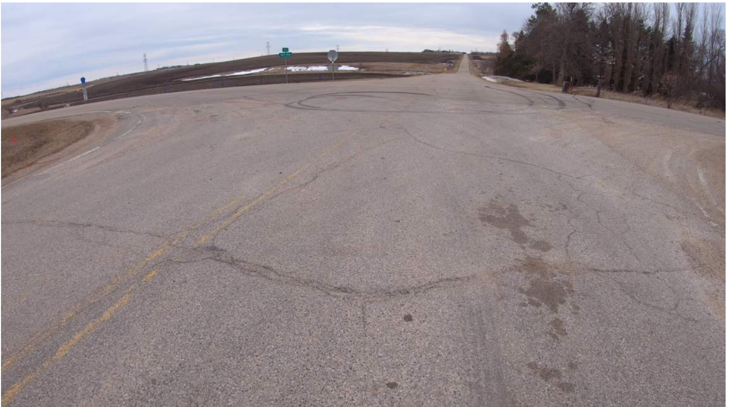
MILE 22 - CCR 20 - Intersection 464th Ave. Time 4:11 on Pre Segment B2
