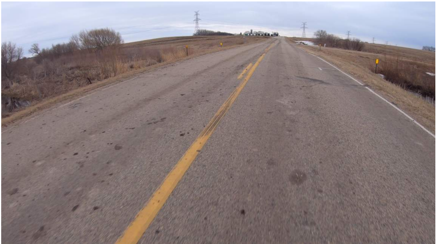
MILE 23 - CCR 20 - Intersection 465th Ave. Time 6:14 on Pre Segment B2
