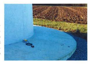
Figure 4.8-1: Vibration measurement point MPA at the tower foundation of WT 5. Photo: Wölfel company
