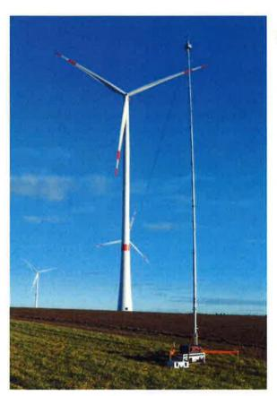
Figure 4.6-1: Wind turbine WT 5 in surroundings used for agricultural purposes. In the foreground you can see the 10 m high wind measurement mast. Photo: Wölfel company
