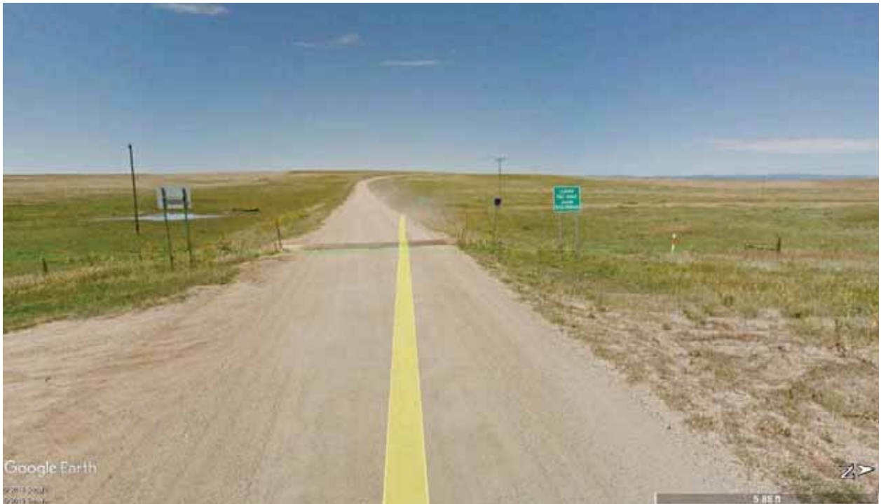
Figure 9, View of Riverside Road from Solar Park Site, Facing West
