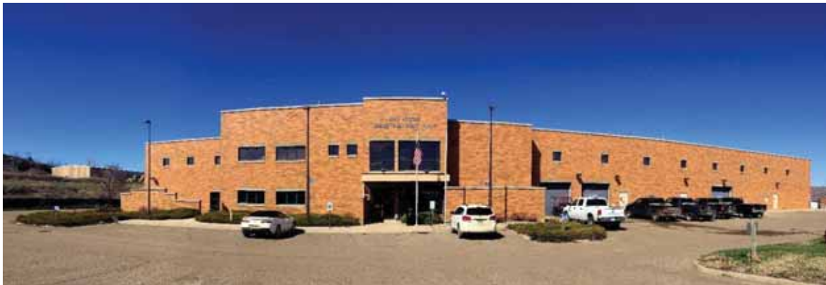
Figure 5, Mni Wiconi Water Treatment Plant
