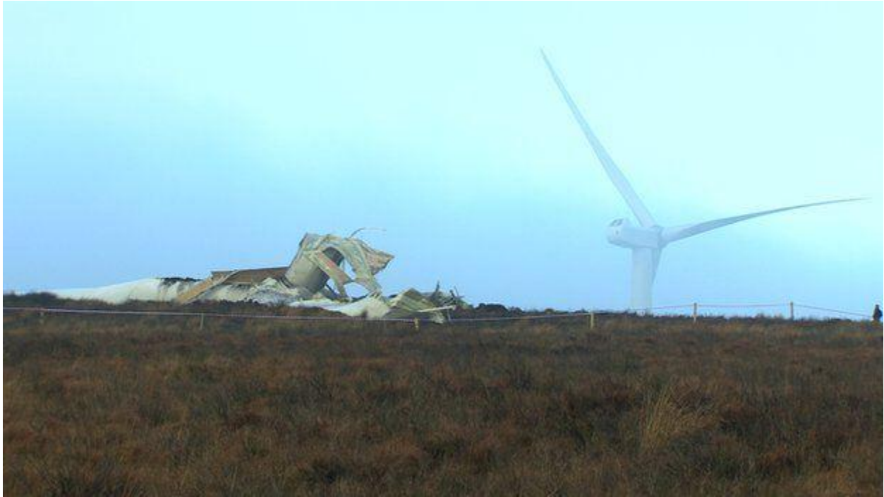
Northern Ireland, Screggagh Wind Farm: Debris from the turbine was scattered across the mountainside and a large spike was impaled in the earth several hundred meters from the turbine site.
