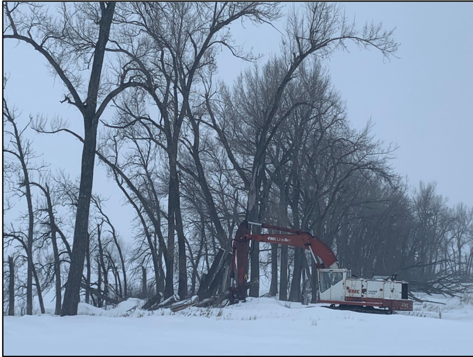
Photograph A-7: View of shelterbelt, excavator, and tree removal along south end of shelterbelt from 172 nd Street, facing north.
