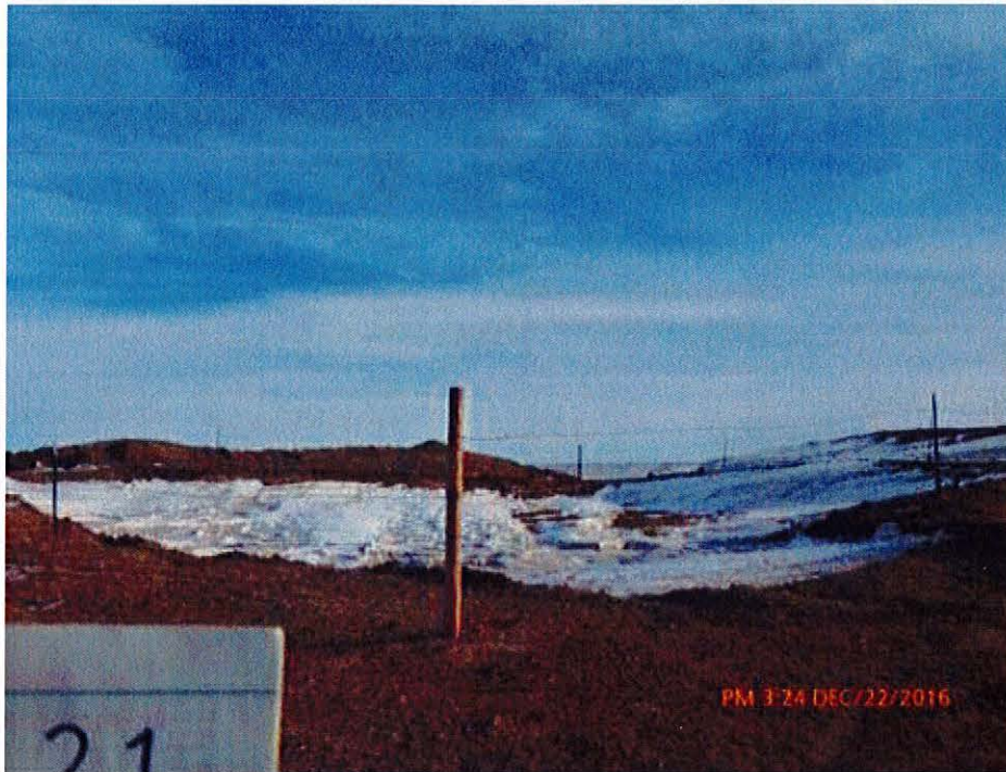
Figure 5 Excavation at turbine T21
