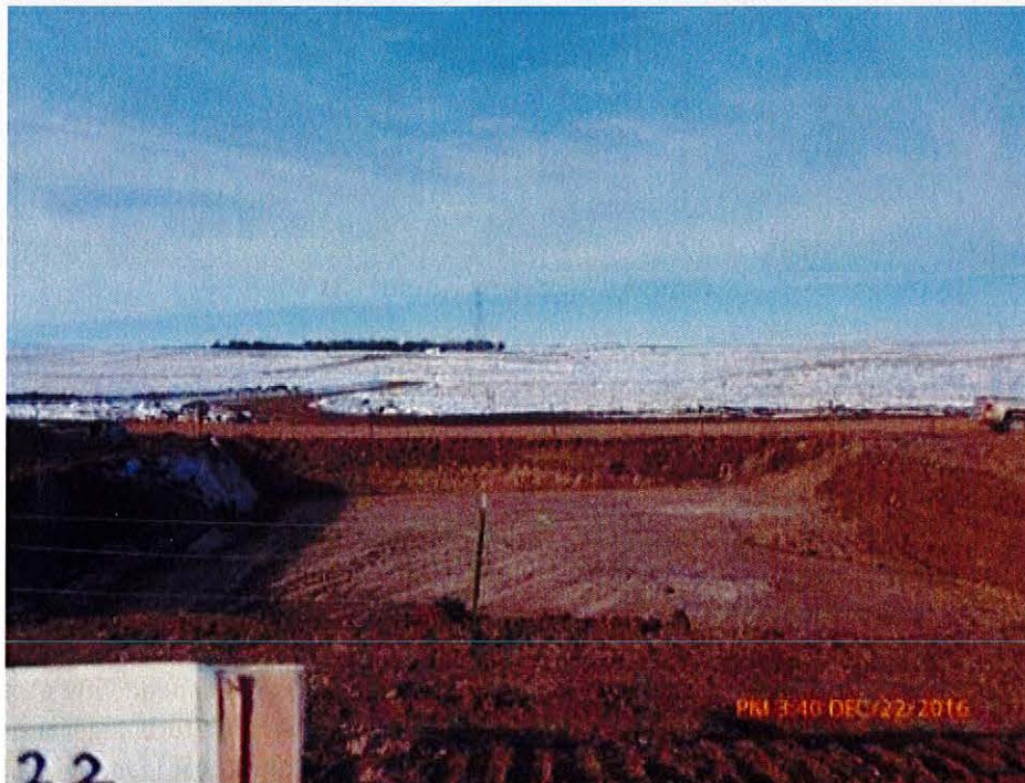
Figure 3 Turbine access road near T22
