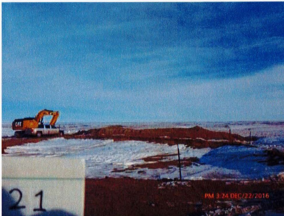
Figure 1 Excavator near T21
