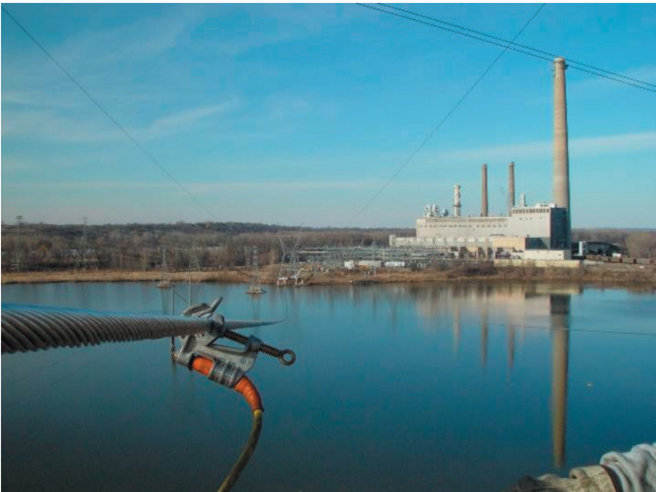
Ceramic Composite Conductor on 115 kV Line
