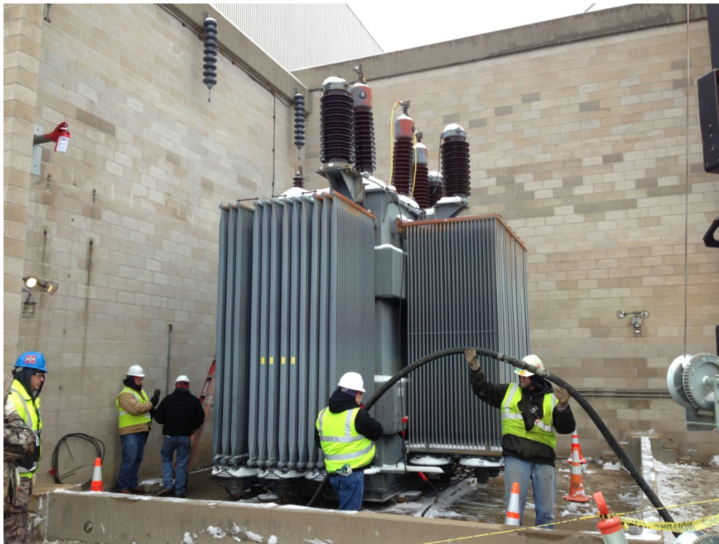
Existing 1R Transformer Removal
