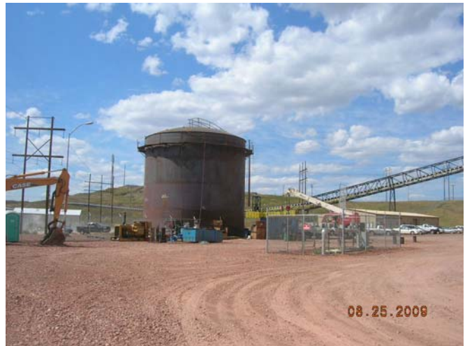
Service Water Storage Tank
