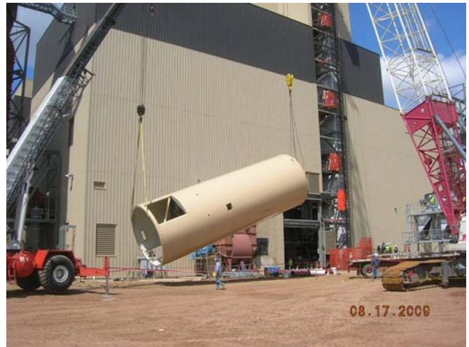
PAC Silo Installation
