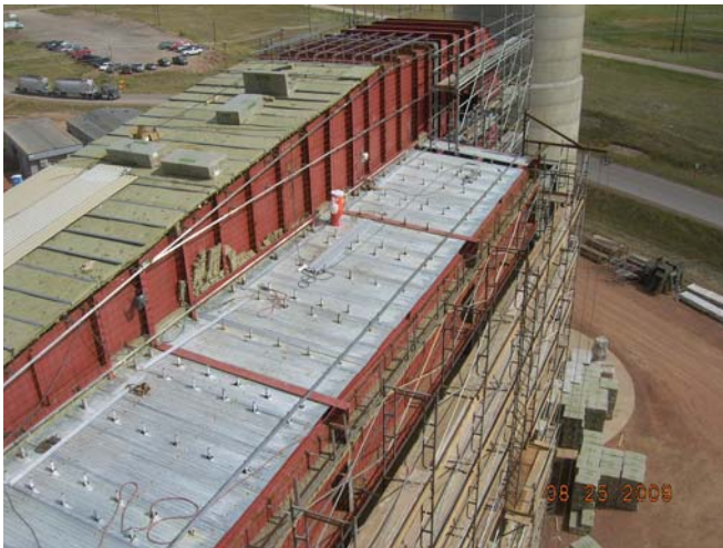
Baghouse Insulation and Lagging
