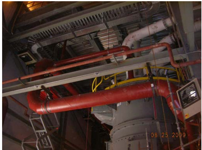
Pulverizer Seal Air Piping
