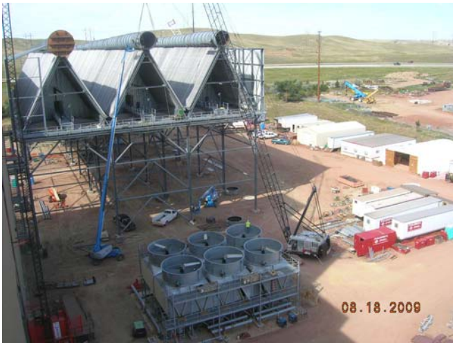
ACW/ACC Erection Progress
