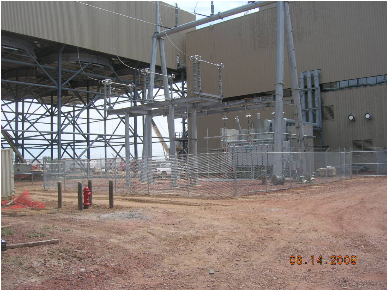
Transformer Yard Progress
