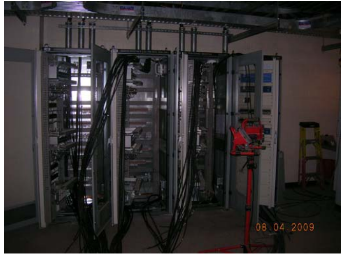
Relay Protection Cabinet
