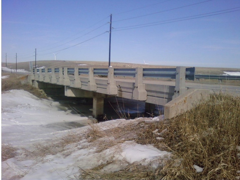
486 th Avenue Bridge – 0.8 miles south of 207 th Street – 73x32' bridge deck
