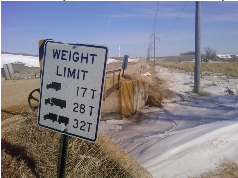
207 th Street Bridge – 0.6 miles east of 484 th Avenue - Load limit sign
