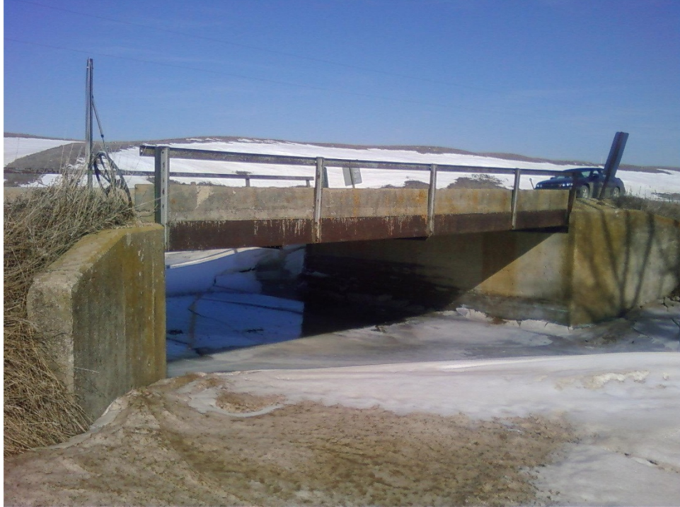
207 th Street Bridge – 0.6 miles east of 484 th Avenue – 29x23' bridge deck
