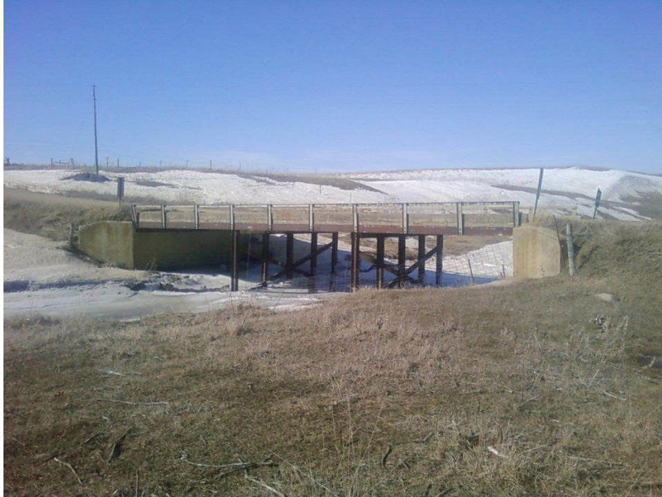
207 th Street Bridge – 0.2 miles east of 484 th Avenue – 54x24' bridge deck
