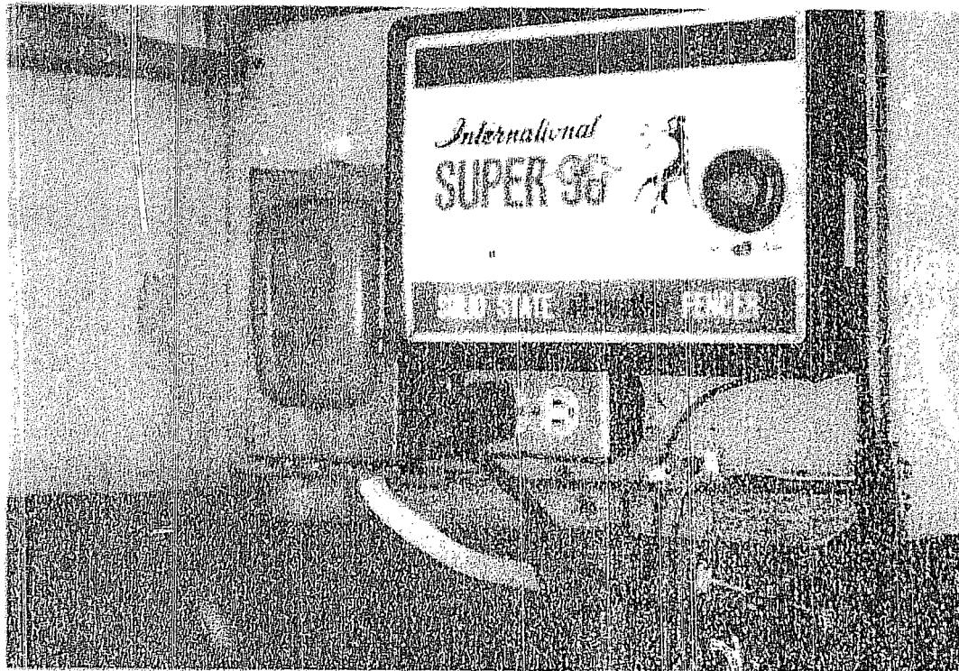
A wire apparently extends from the meter underground to a post about 100 Feet South of the meter. A switch and outlet are mounted on this post.
