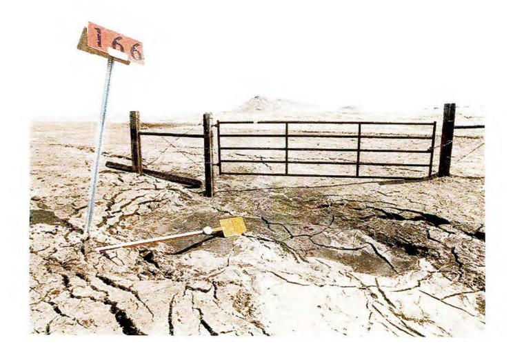
Janelle Reiger walks on a concrete creek crossing damaged during installation of the Bison high pressure gas pipeline in southeast Montana 04/12/2011
