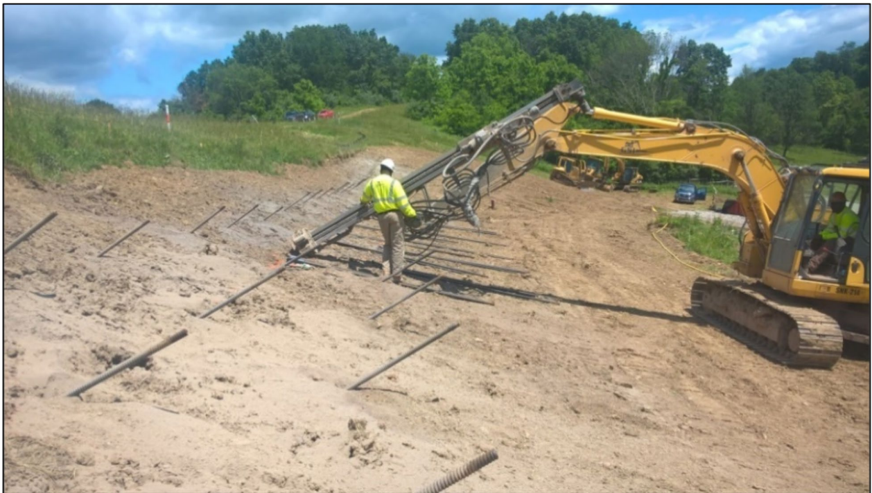
Figure 8-4. Installation of soil nails combined with site regrading to stabilize a landslide downslope of a pipeline ROW
