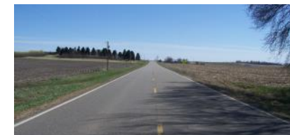
Minor Collector - Co. Hwy. 143
