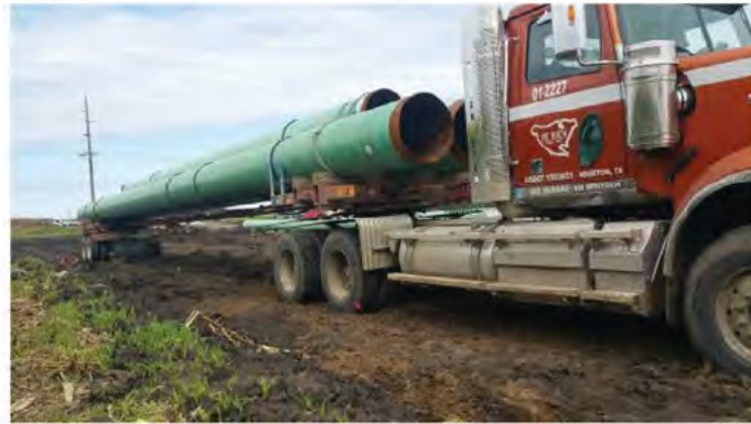
Semi-trailer truck with three pipes (each pipe was 24.4 m long, 0.76 m outer diameter, and 9.5 mm wall thickness).
