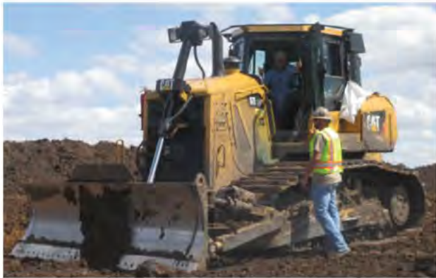
Caterpillar D7E bulldozer. Fully loaded weight = 256 kN. Each track had a nominal track contact length of 3.02 m and a width of 0.76 m.
