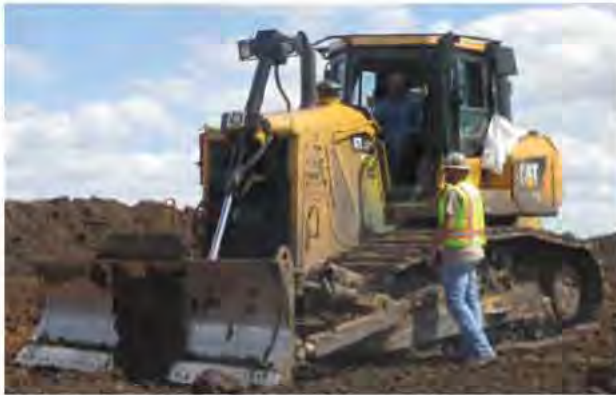
Caterpillar D7E bulldozer. Fully loaded weight = 256 kN. Each track had a nominal track contact length of 3.02 m and a width of 0.76 m.
