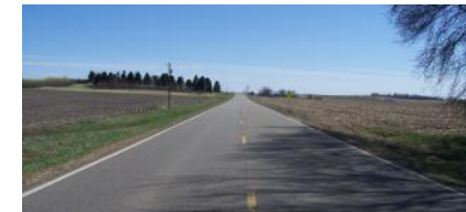
Minor Collector - Co. Hwy. 143
