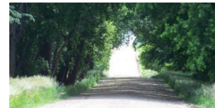
Local Roads - East 264th Street
