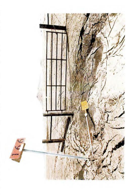
Janelle Reiger walks on a concrete creek crossing damaged during installation of the Bison high pressure gas pipeline in southeast Montana 04/12/2011
