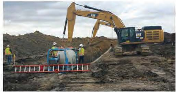
Caterpillar 349F hydraulic excavator. Fully loaded weight = 522 kN. Each track had a nominal track contact length of 5.36 m long and a width of 0.76 m.
