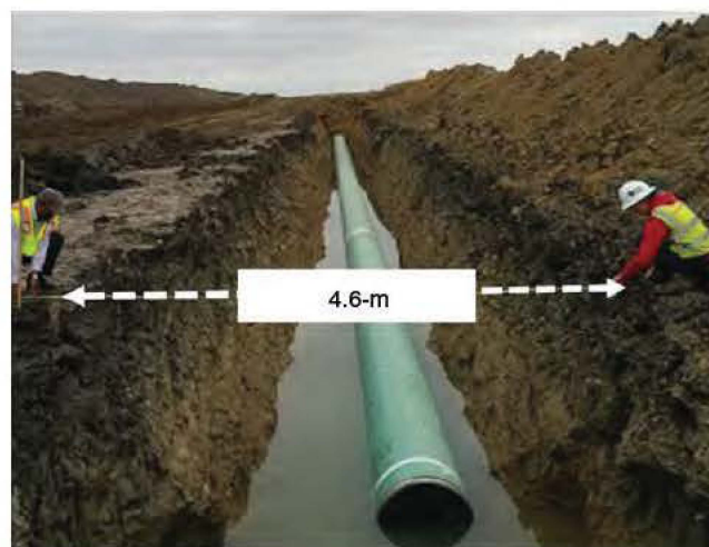
FIGURE 1 Right-of-way pipeline construction heavy equipment—Caterpillar pipe liner PL 87, Caterpillar 349F hydraulic excavator, Caterpillar D7E bulldozer and semi-trailer truck with three pipes (a). The excavated trench for the pipe and the stockpiled subsoil adjacent to the pipe (b). At the experimental site, the pipe trench width was approximately 4.6 m [Colour figure can be viewed at wileyonlinelibrary.com ]
