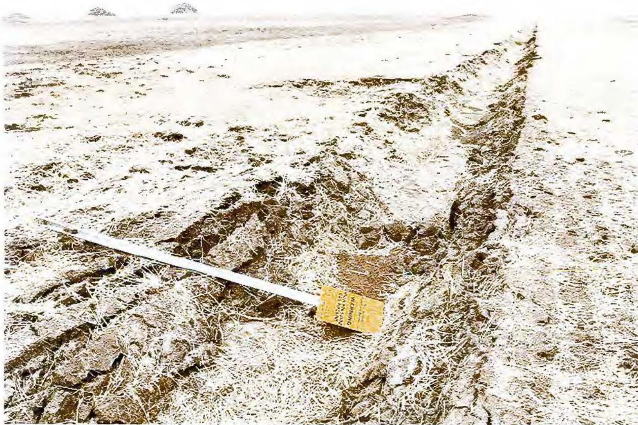
One sign has fallen while another leans in the soft soil on the Bison high pressure gas pipeline right of way in southeast Montana 04/12/2011
