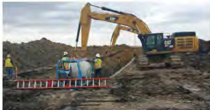
Caterpillar 349F hydraulic excavator. Fully loaded weight = 522 kN. Each track had a nominal track contact length of 5.36 m long and a width of a 0.76 m.
