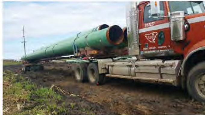
Semi-trailer truck with three pipes (each pipe was 24.4 m long, 0.76 m outer diameter, and 9.5 mm wall thickness).
