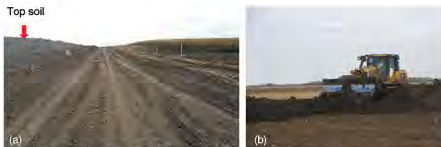
FIGURE 1 (a) Topsoil pile adjacent to the ROW zones. (b) The top soil was replaced by a Caterpillar D7E bulldozer after the exposed subsoil was tilled. The Caterpillar D7E fully loaded weight was 256 kN. Each track had a nominal track contact length of 3.02 m and a width of 0.76 m (Tekeste et al., 2019) [Colour figure can be viewed at wileyonlinelibrary.com ]
