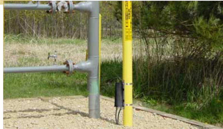
SSD – Solid State Decoupler
