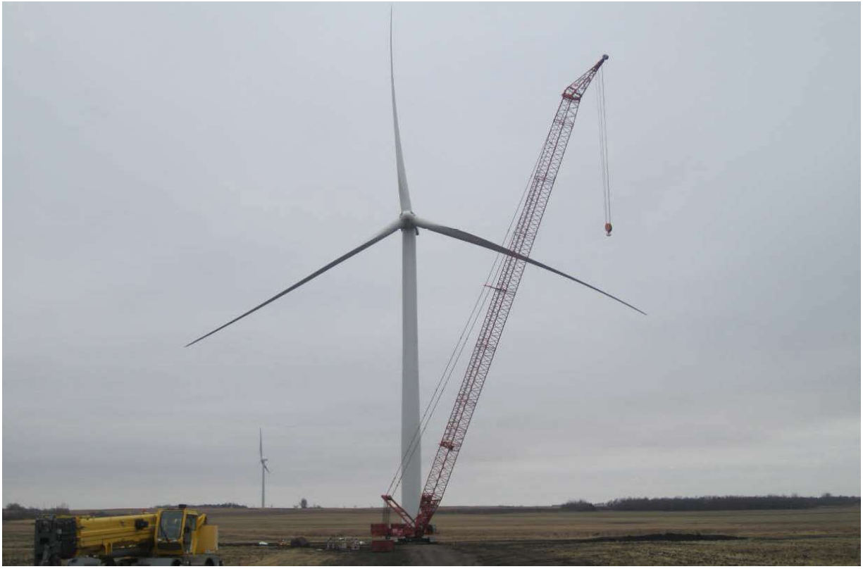
Photo: Wind tower construction west of Waverly.
