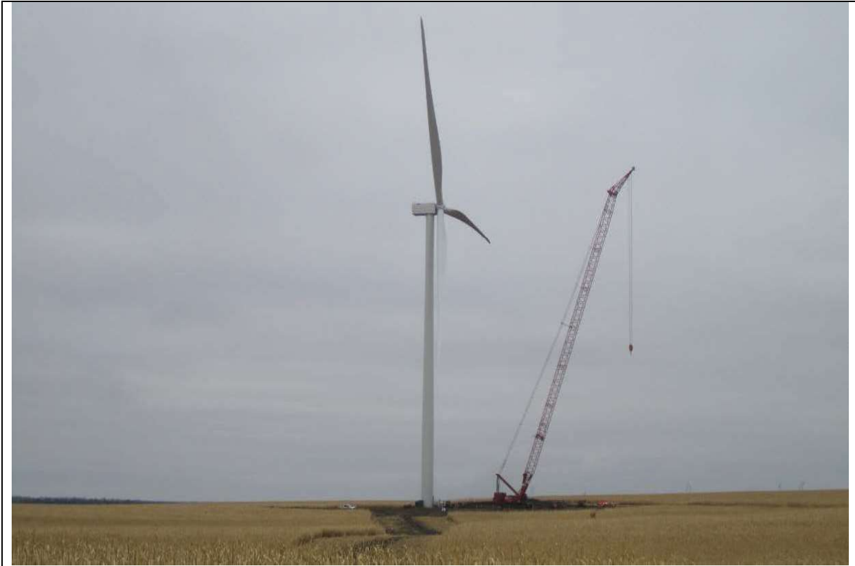
Photo: Wind tower construction west of Waverly
