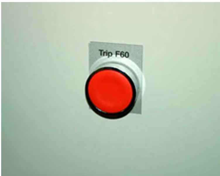
Picture 6 The trip F60 button (pos. 5, Figure 1)
