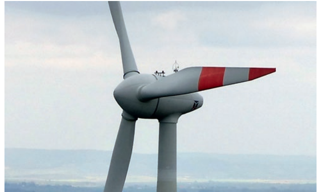
Figure 4-2: Model type WT 2, Enercon E-66
