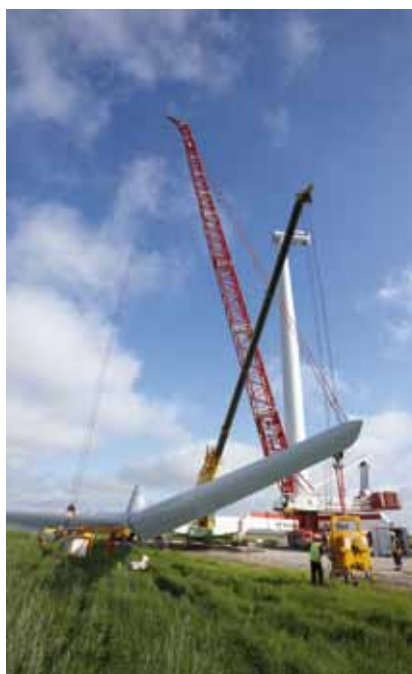
The Vattenfall electricity company, which is the largest owner of Danish onshore wind turbines, was also responsible for the largest project under the scrapping scheme at Nørrekær Enge, where 77 older wind turbines were replaced with 13 x 2.3 MW turbines. In the photo, the installers are setting up one of the new wind turbines, which were connected to the grid in 2009.
