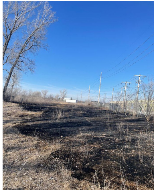
Encroachment fire example near a substation
