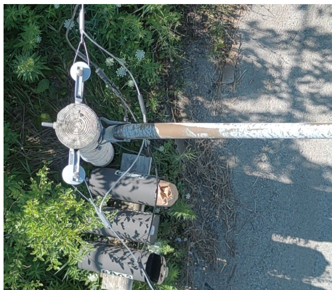
Example of Image from a Drone Inspection
