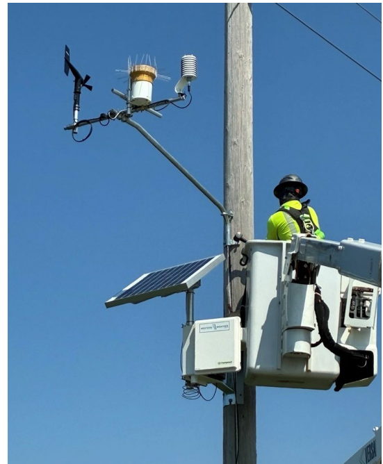
Example of weather station being installed
