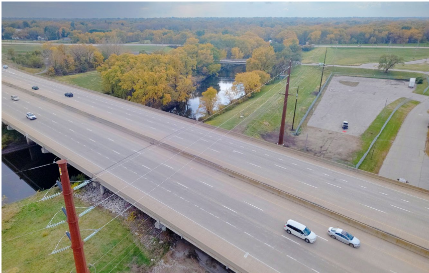
Example of Interstate Containment/Non-Wood Pole Installations
