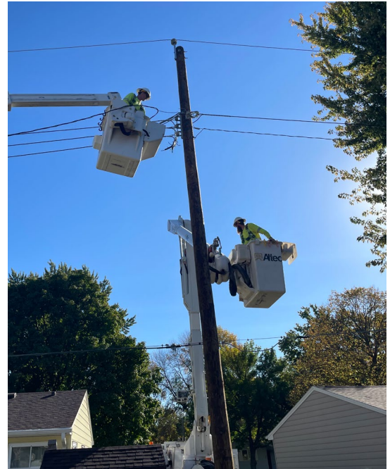
Example of pole replacement
