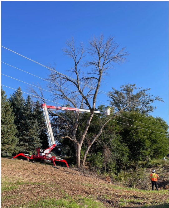
Example of Vegetation Management Work
