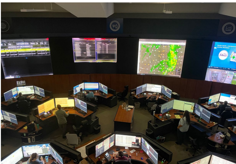
System control – where remote de-energizations occur
