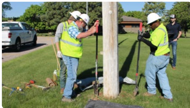
Figure 15: Example pole inspection
