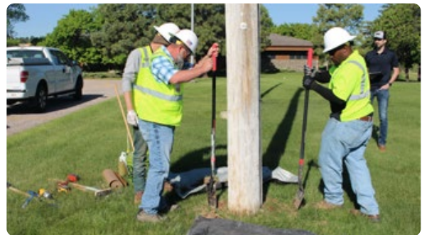
Figure 15: Example pole inspection
