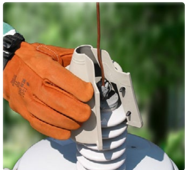
Figure 18: Example of wildlife guards on overhead equipment
