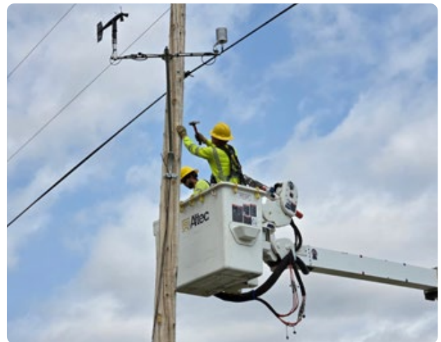
Figure 20: Black Hills Energy crew installs a weather station
