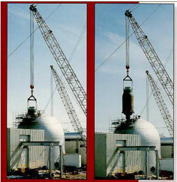
*When crews installed the reactor assembly in the Pathfinder's containment building, the optimism surrounding the project was palpable. The superheater's job in the core of the reactor was to make hot steam even hotter. Steam produced and heated to 489 degrees in the boiler region of the reactor was designed to be channeled through uranium dioxide fuel tubes in the superheater, where its temperature would be raised to 825 degrees.*
