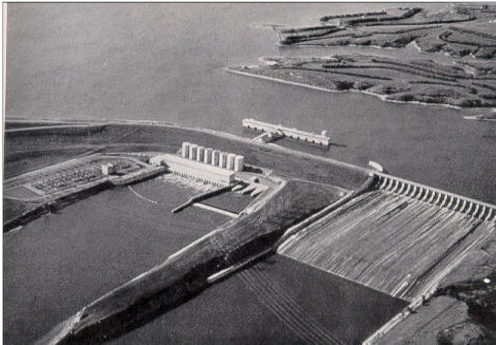
*The Fort Randall Dam with eight turbine generators can produce up to 320 megawatts of electric energy. It is one of the eight major hydroelectric sources located along the Missouri River (four in South Dakota) in the Upper Midwest.*
