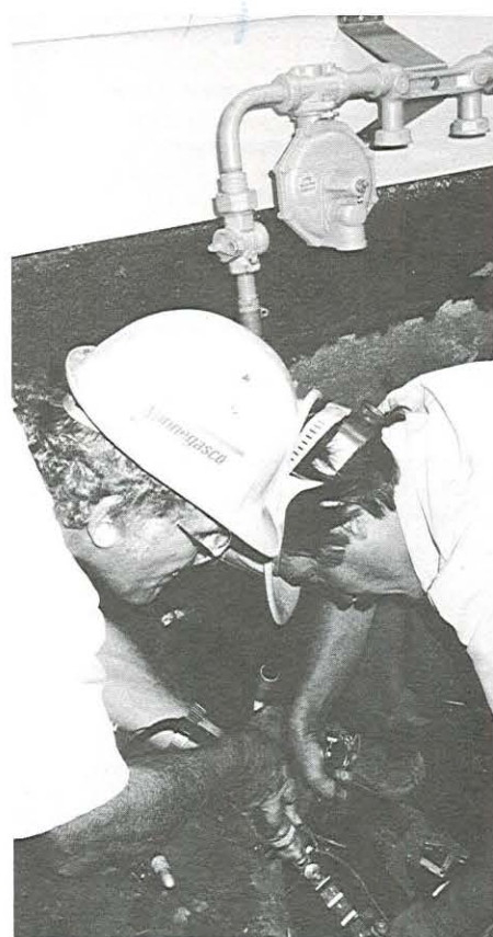
Distribution Foreman Bill Keiser and Distribution Mechanic Bill Warren install a service line in Sioux Falls.
