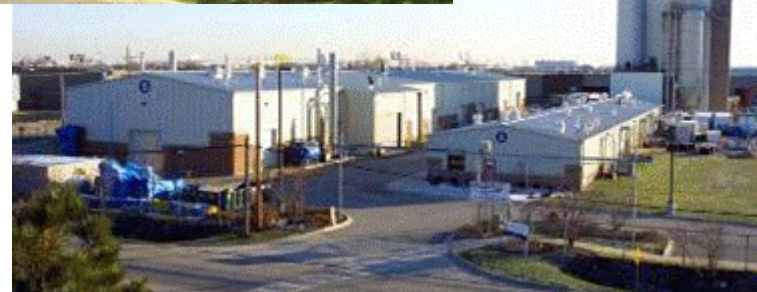
Energy & Environmental Technology Center
