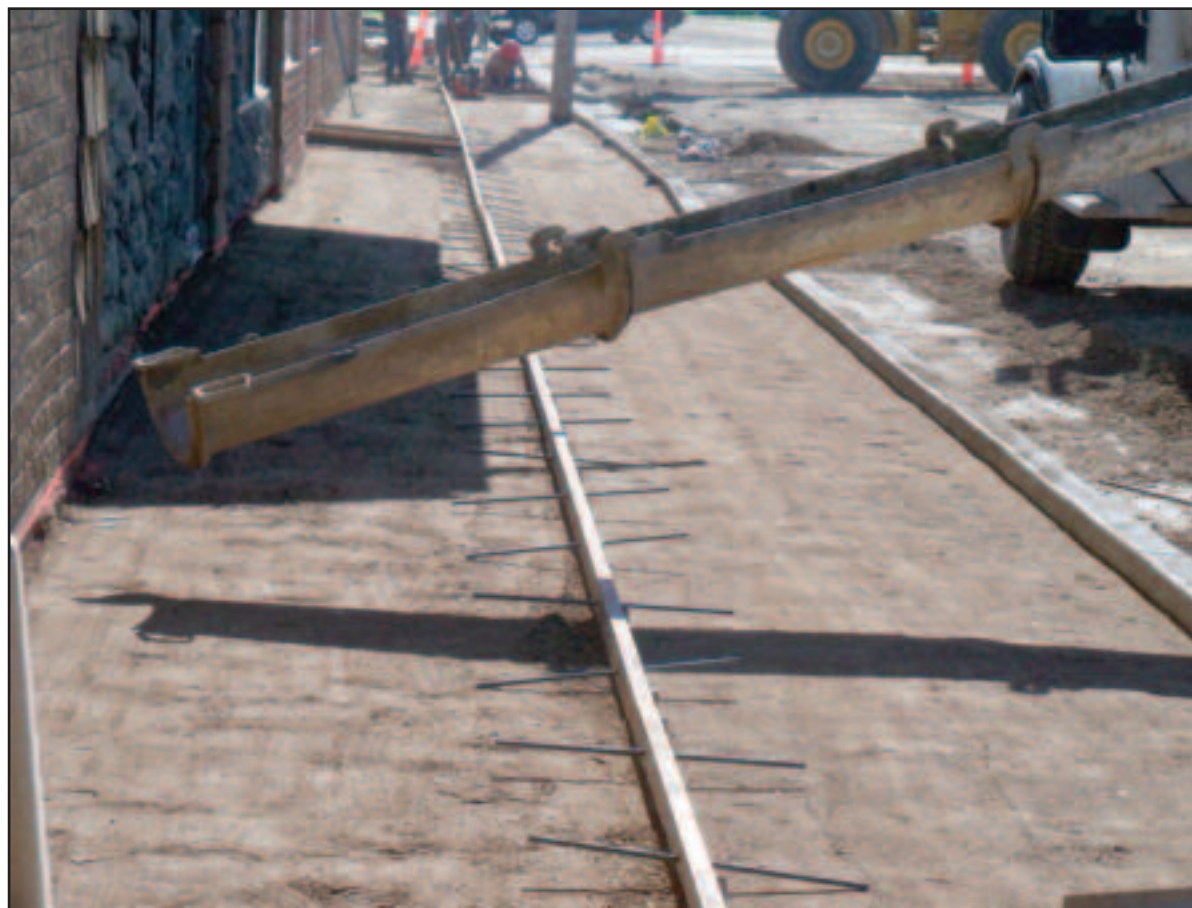
Hoff's Ready Mix of Lemmon delivered cement for the new sidewalk, curb & gutter.
