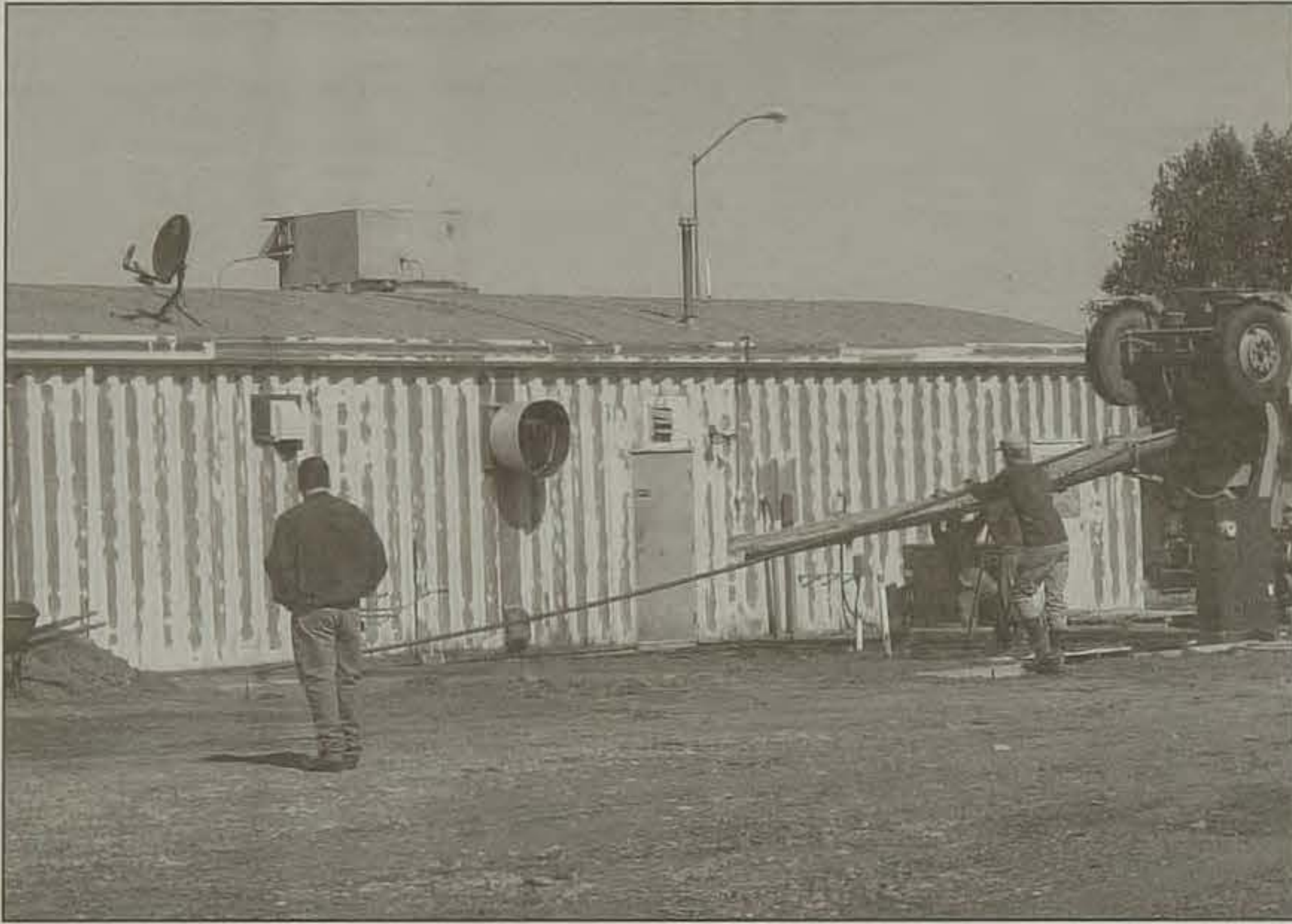
Ryan Maher, owner of Sparky's Cafe in Isabel, watches as crews pour concrete in the back of the building recently. Sparky's is planning to expand its kitchen this summer.
